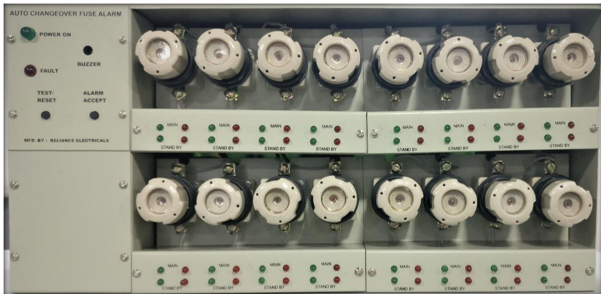
16 Fuse Bottle/ 'D' Type FUSE AUTO CHANGEOVER SYSTEM (FACS)
